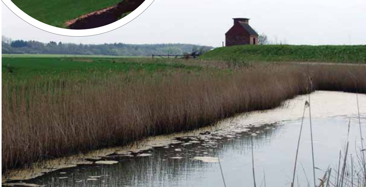
Pumpehus, Kahr Holme Digelag
