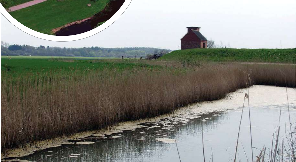
Pumpehus, Kahr Holme Digelag
